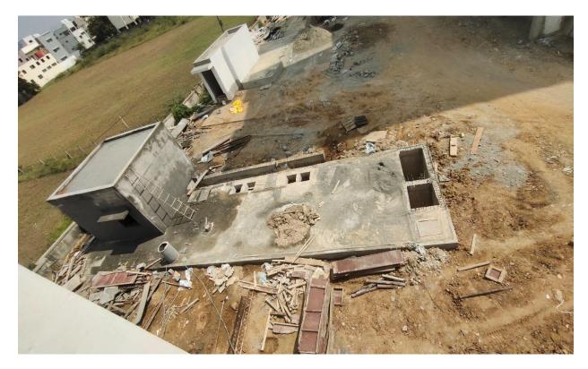
**U.G Sump 2 (Near D Block)** – All RCC works completed. Pump room work completed. Internal Water proof plastering works on progress.
