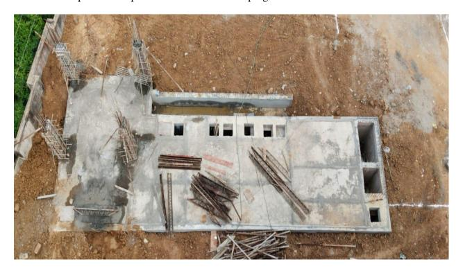
**U.G Sump 1 (Near D Block)** – Base Slab RCC 95% completed. Sump wall & Top Slab Concrete 100% completed. Inner plastering works on progress.
