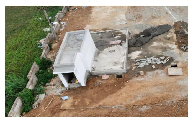
**U.G Sump 2** – Base Slab RCC 95% completed. Sump wall Concrete completed. Shuttering & Barbending works for Top Slab completed.
