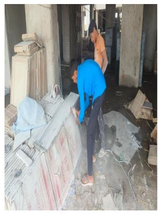
**Block A2:** Laying of bathroom & toilet floor tiles, vitrified tiles on progress.
