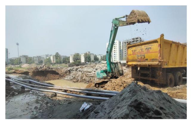
**External Sewerage Lines**: Laying of External Sewage line & construction of Chambers around D2 & D3 Block
