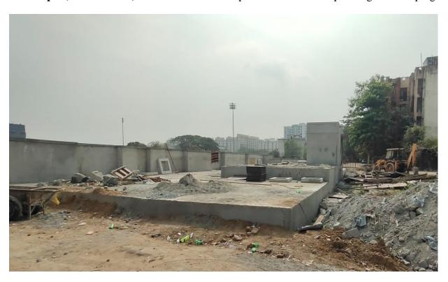
$\begin{tabular}{ll} \textbf{U.G Sump 2 (Near D Block)} - \textbf{All RCC works completed. Pump room Inner plastering \& Internal Water proof plastering works on progress. \end{tabular}$
