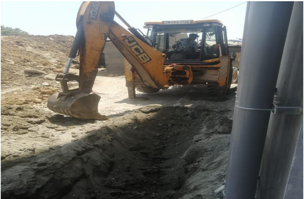
Excavation for laying of Sewer lines in C1-Block on progress.
