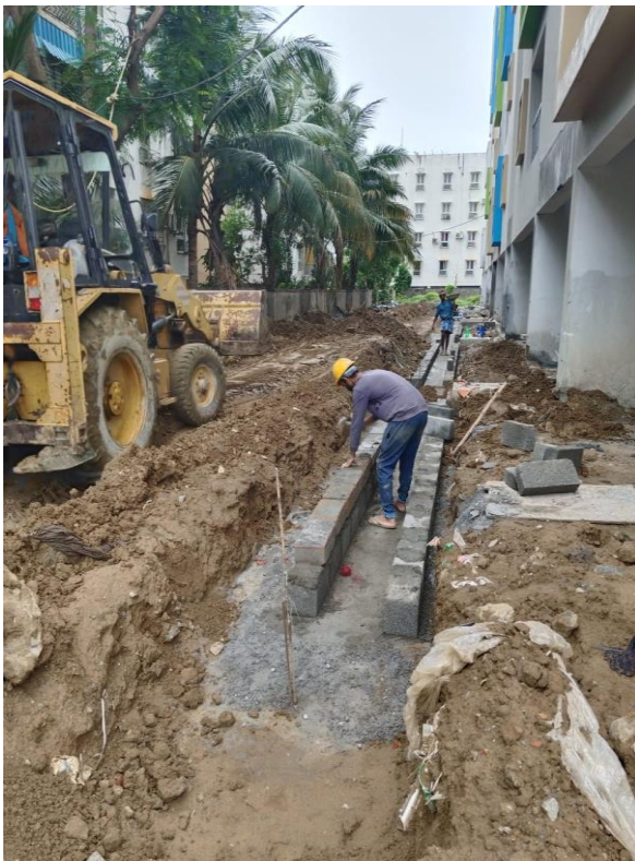
B1- BLOCK WEST SIDE
