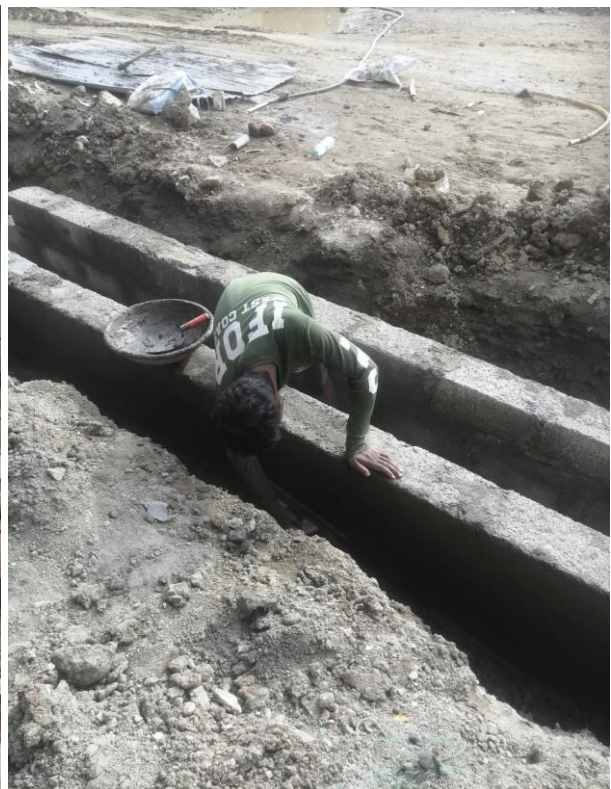
C3-BLOCK WEST SIDE
