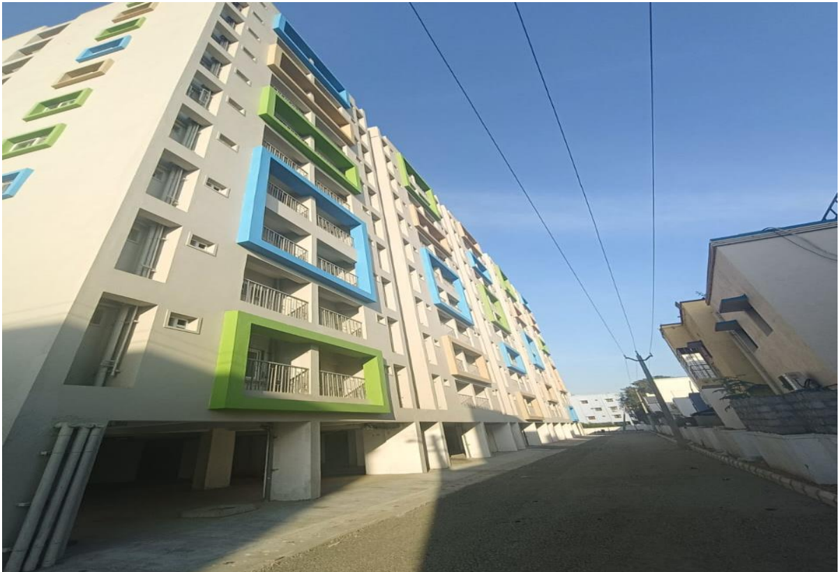
Block A2 – South side Elevation & Road work
