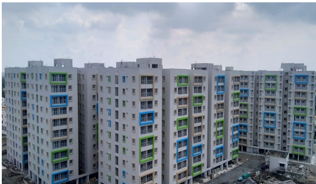
View of C1,C2 ,C3 West Side & A1 Block North Side Elevation
