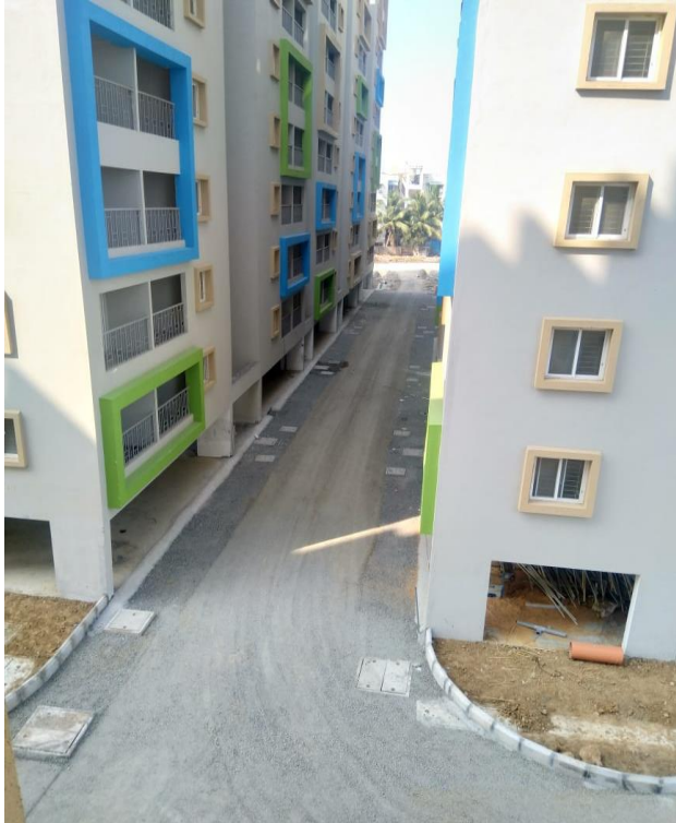
Road between C1 & C2
