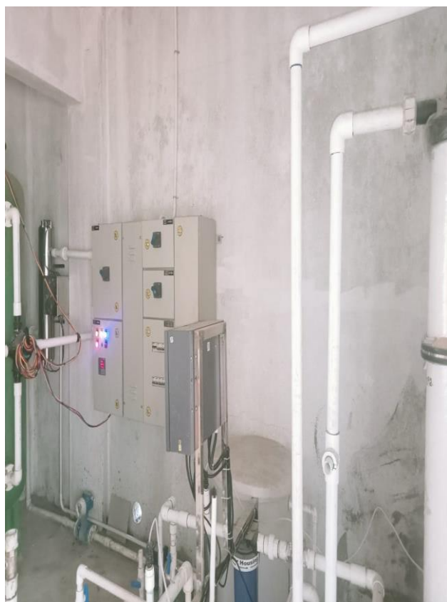
STP-2 – Erection completed & dry testing of components completed
