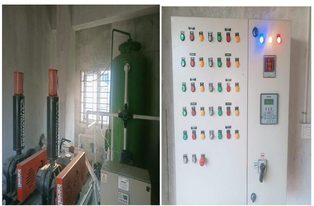
STP-2 – Erection completed & testing for Commissioning on process
